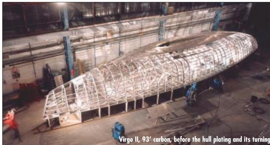
Virgo II, 93' carbon, before the hull plating and its turning
